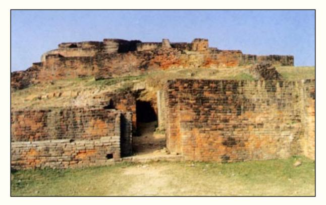
**Plate 27. Sravasti**. The Angulimala *stupa* at Mahet, showing the opening of a tunnel cut through its base for drainage. **RETURN**
